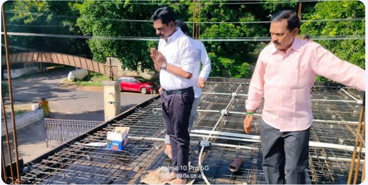
Roof Construction Puja for new building in the college campus on September 6, 2025
